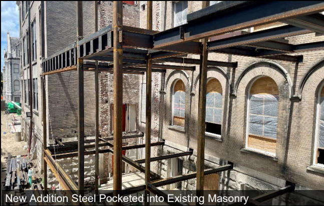
New Addition Steel Pocketed into Existing Masonry
