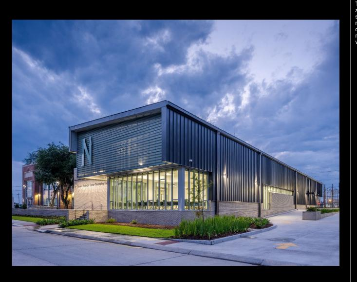
The campus façade uses perforated and corrugated metal scrim and standing seam metal panels, mimicking the community face. The conference room, located under the roof cantilever, offers expansive views of the campus.
