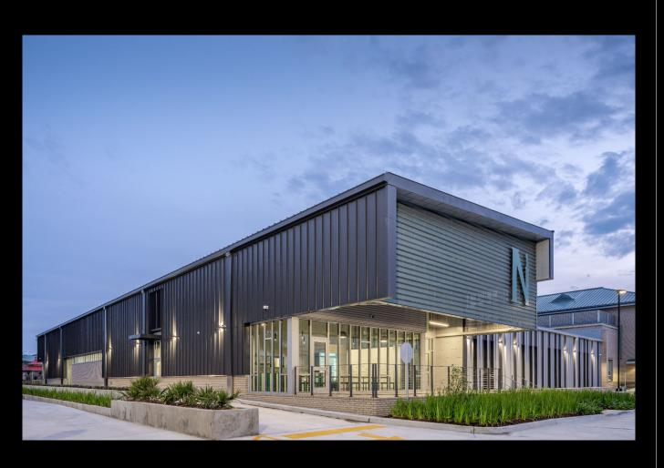
The community façade features a welcoming entry with an outdoor covered dining space. The east façade is shaded with a perforated, corrugated metal scrim, providing filtered light, transparency, and ventilation. The café includes a drive-up window, separated from the parking area by a landscaped planter.
