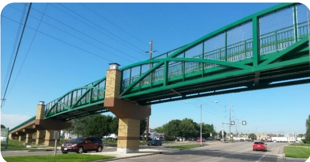
Pedestrian Overpass of County PD/McKee Road for the Military Ridge Trail. The overpass provides a critical grade separated safe crossing for users of the Military Ridge Trail.
