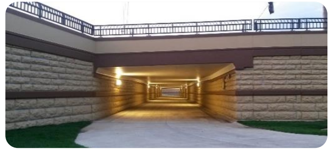
One of the 4 critical neighborhood links, this underpass (8 feet tall, 20 feet wide, 323 feet long).
