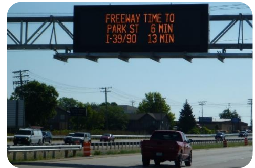
New DMS along the Beltline provided travel times for alternative routes to drivers throughout construction.
