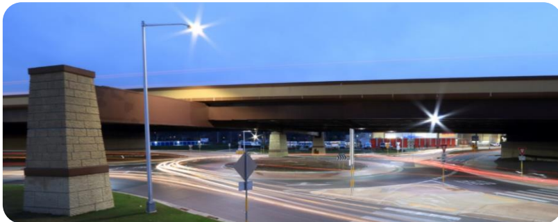
Straddle Bent Bridge over Local Road Roundabout.
