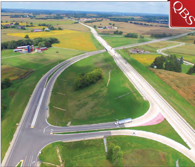
An innovative design shaped like a jug handle minimizes crashes and facilitates traffic flow between two major highways.
