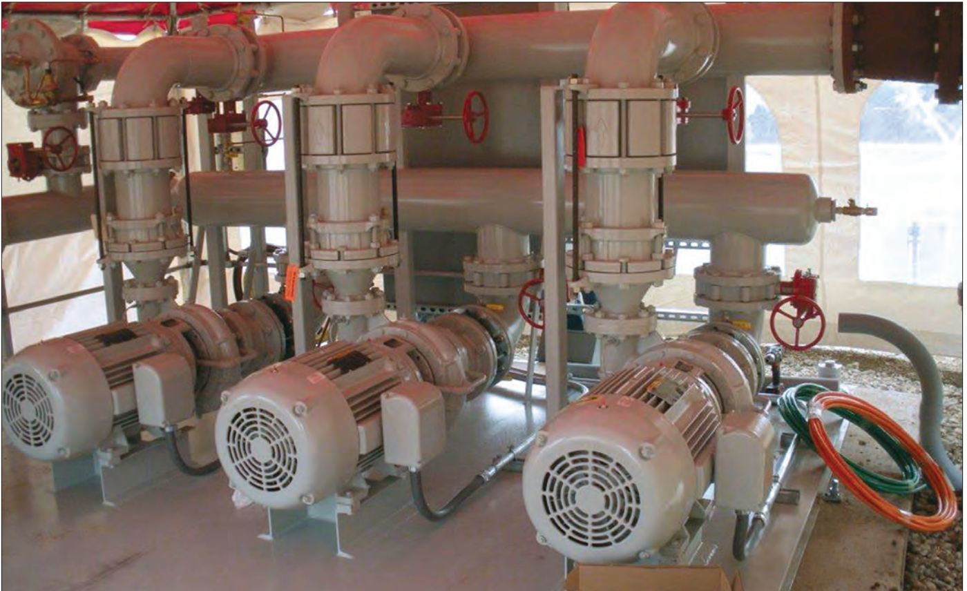
TOP: The temporary station was able to keep up with the demands of supplying 1.5 million gallons daily and no complaints were received. BOTTOM RIGHT: The pump was located in the median which allowed efficient operation and no disruption of traffic.
