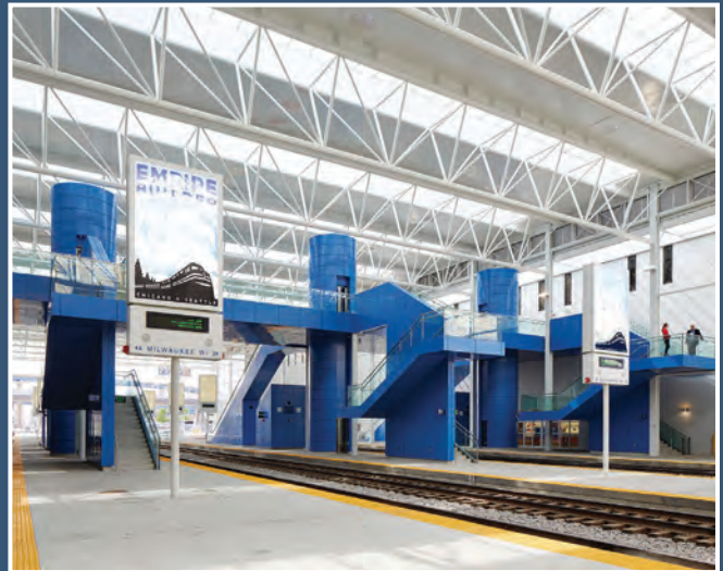
Milwaukee Intermodal Station Passenger Train Concourse (with Alfred Benesch & Company, project team leader)
