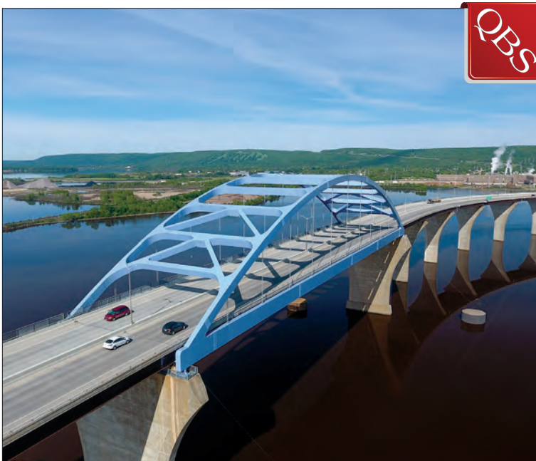
The rehabbed structure connects Superior, WI and Duluth, MN and serves over 20,000 vehicles a day.
