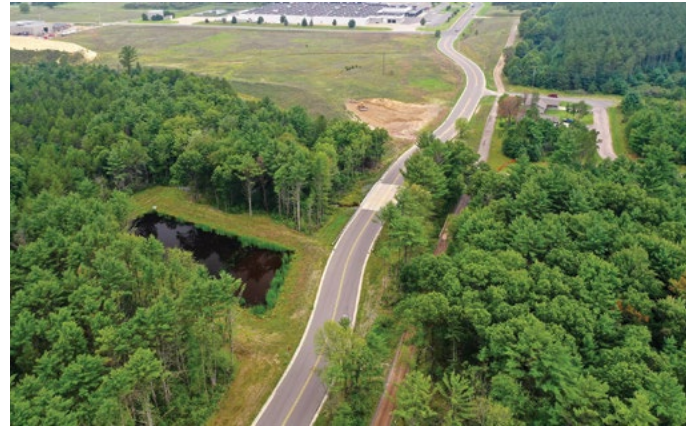
The road twists and turns slightly to minimize environmental impacts.
