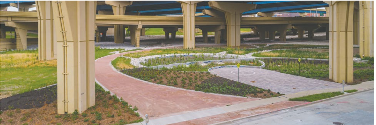
Marquette Interchange Green Infrastructure Project — Milwaukee Metropolitan Sewerage District — Milwaukee, WI
