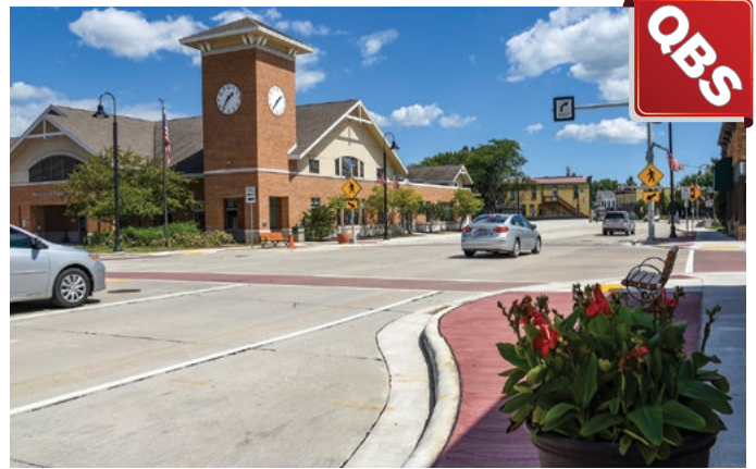
Curb bump outs and high-visibility crosswalks promote pedestrian safety.
