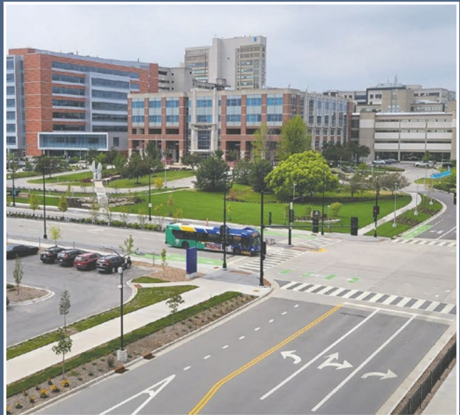
87th St. Reconstruction | Milwaukee Regional Medical Center
