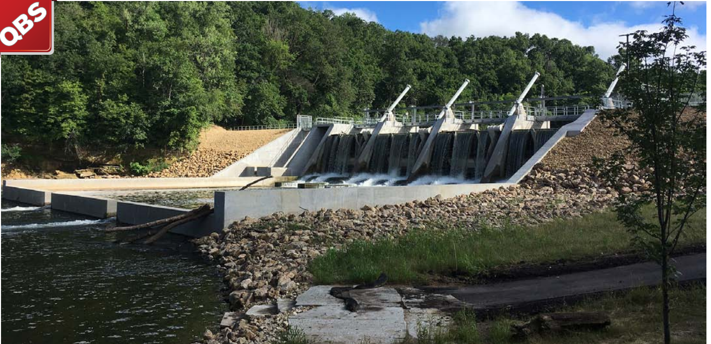
The new control gates allow proper water flow in addition to regulating temperature and sediment discharge.
