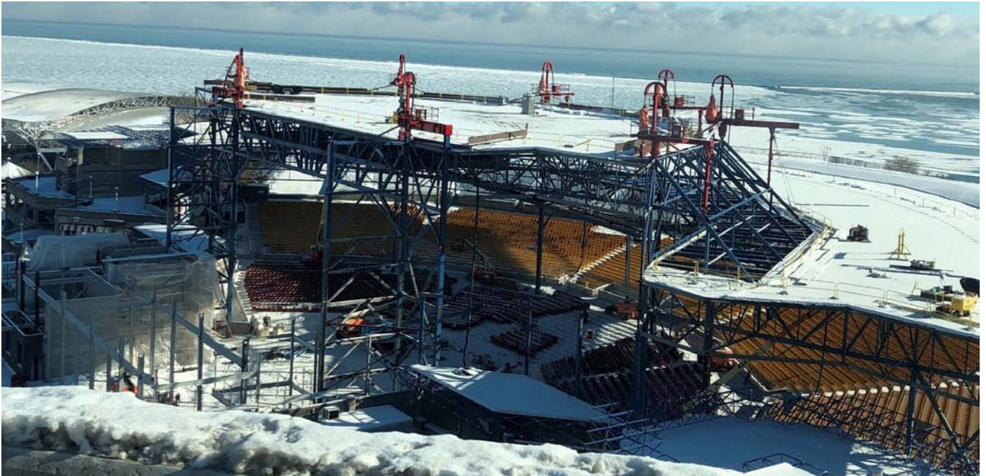
A 300-ton center portion of the roof was lifted in the middle of winter to stay on schedule.
