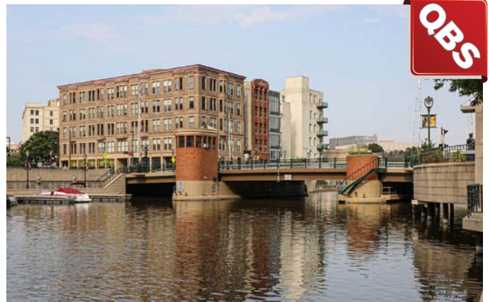
By replacing the mechanical components, the lift bridge will be able to function as intended to let boats pass underneath.
