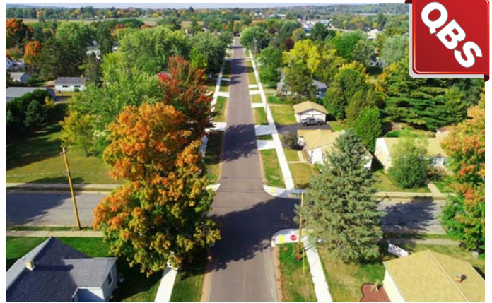
The new design features of the road provide a safer design and set a standard for other roads in the city.
