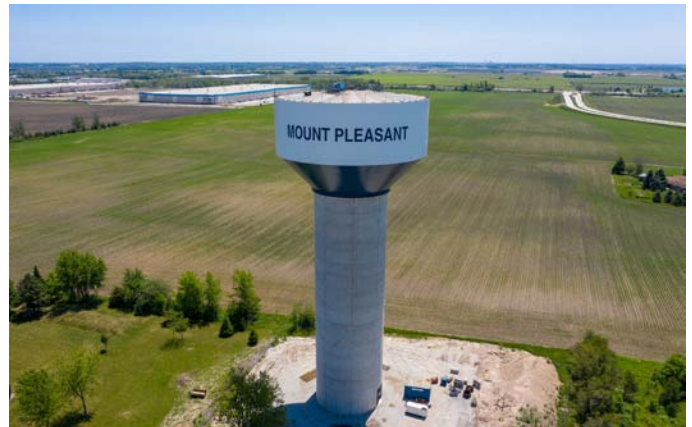
A new water tower supports the water infrastructure below and signposts the development for the village.
