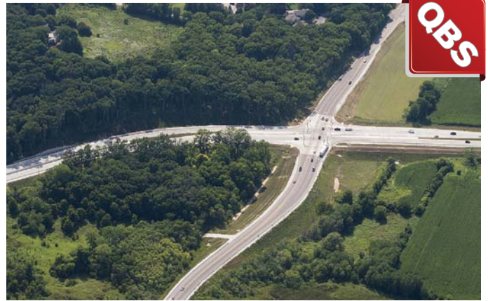
The new widened roads and modern intersections provide room for the community's future growth.
