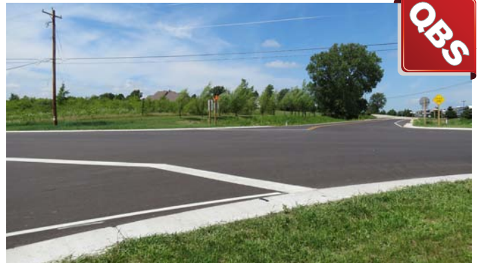
The new two-way stop at this intersection is safer than the previous intersection and prioritizes traffic on the busiest road.
