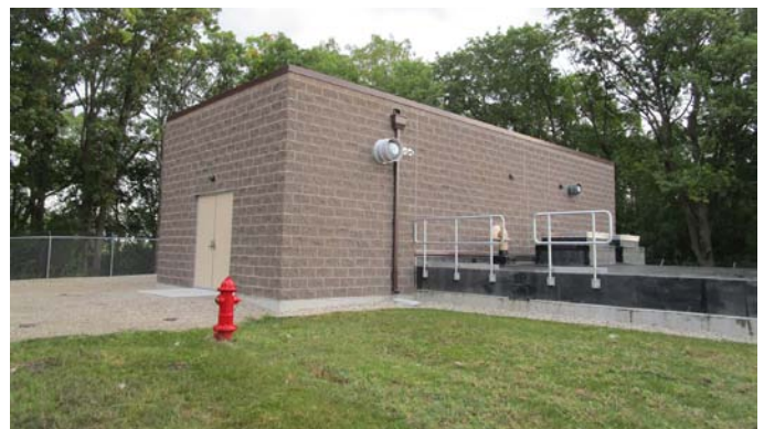
The new wellhouse was placed on public land, avoiding time-consuming and costly land acquisition processes.
