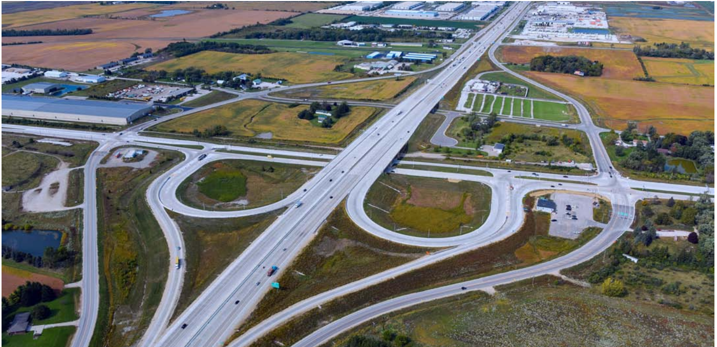
The newly finished corridor quickly and safely moves people and freight between Milwaukee and Chicago.
