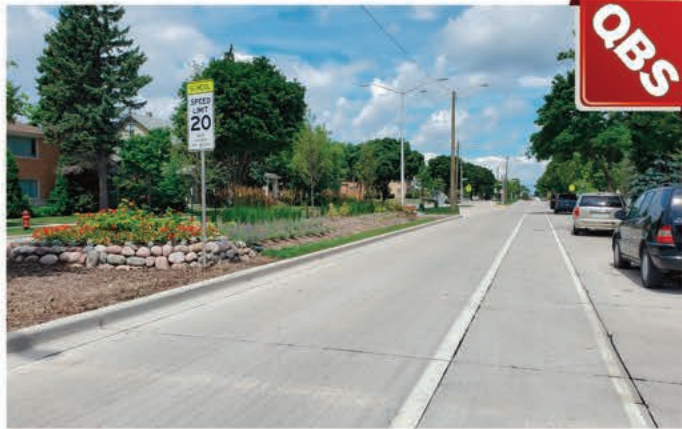
The new road provides more green space, a welcome addition in any cityscape.
