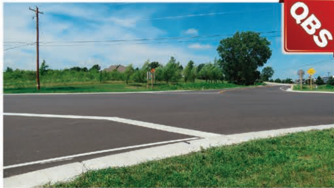
The new two-way stop at this intersection is safer than the previous intersection and prioritizes traffic on the busiest road.
