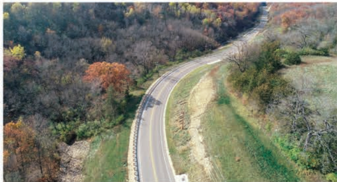
The new road's gentler curves and extensive drainage meet modern design standards and reduce crashes and flooding.
