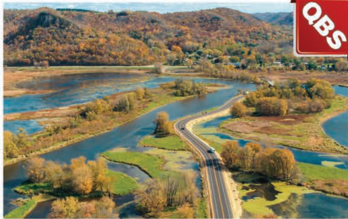
The reconstructed roadway gives users safe access to the beautiful wetlands surrounding the area.
