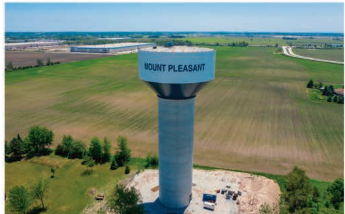
A new water tower supports the water infrastructure below and signposts the development for the village.
