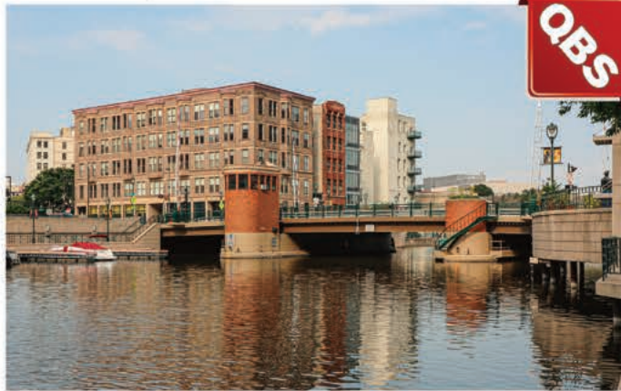
By replacing the mechanical components, the lift bridge will be able to function as intended to let boats pass underneath.
