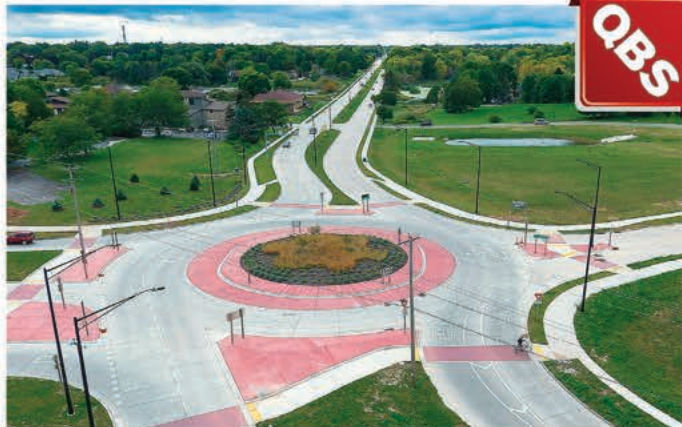
The new multi-lane roundabout is a modern design addition that increases safety at a critical intersection.
