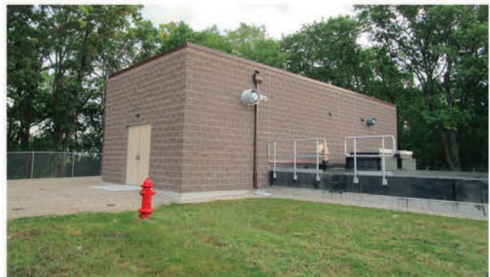
The new wellhouse was placed on public land, avoiding time-consuming and costly land acquisition processes.
