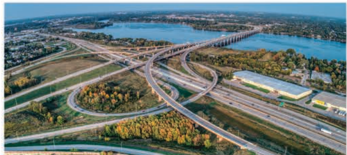
The completed project provides users with quick transit in a fast-growing section of Wisconsin.
