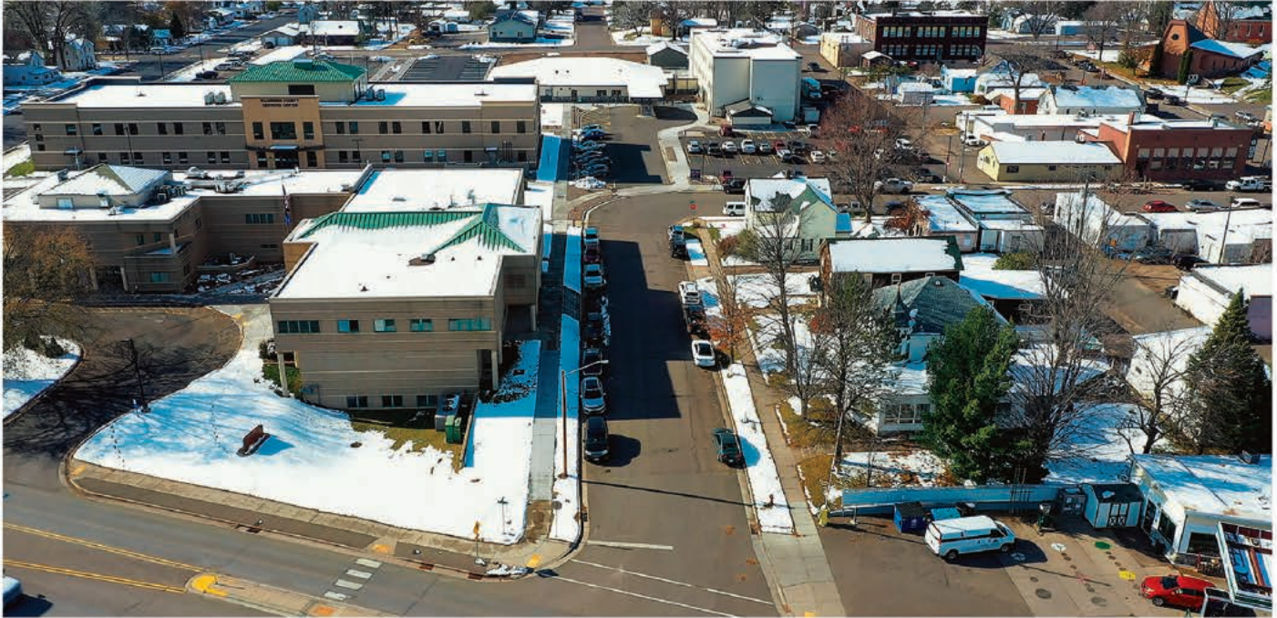
The reconstructed urban roads are safer for multimodal users and keep traffic moving.
