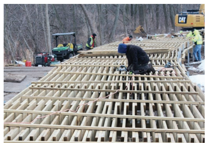
TOP: The final product incorporates viewing areas and an ADA accessible fishing area for all to enjoy. RIGHT: The prefabricated elements could be assembled in any season and greatly facilitated a speedy construction schedule..
