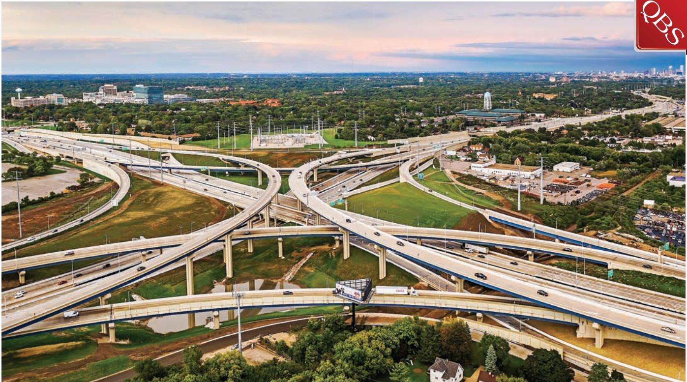
TOP: The final design covers nine miles of interstate and gives Milwaukee a modern infrastructure gateway. BOTTOM: The new design uses longer turning lanes and more right turns to minimize crashes and to keep traffic flowing during rush hour.
