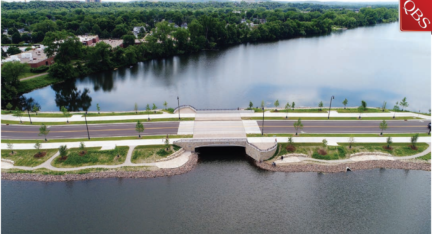
TOP: The new structure has dedicated fishing areas along with bike/pedestrian paths and viewing spots for public use. BOTTOM: The wider footprint of the bridge required removal of old, contaminated sediment from the lake bed and installation of new material for the wider base.
