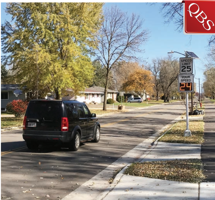
The new design prioritizes multimodal traffic with a large bike/pedestrian lane and digital street signs to reduce car speeds.
