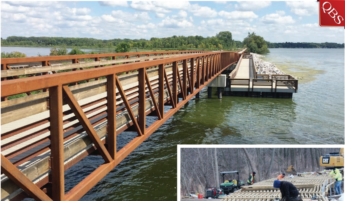
TOP: The final product incorporates viewing areas and an ADA accessible fishing area for all to enjoy. RIGHT: The prefabricated elements could be assembled in any season and greatly facilitated a speedy construction schedule..
