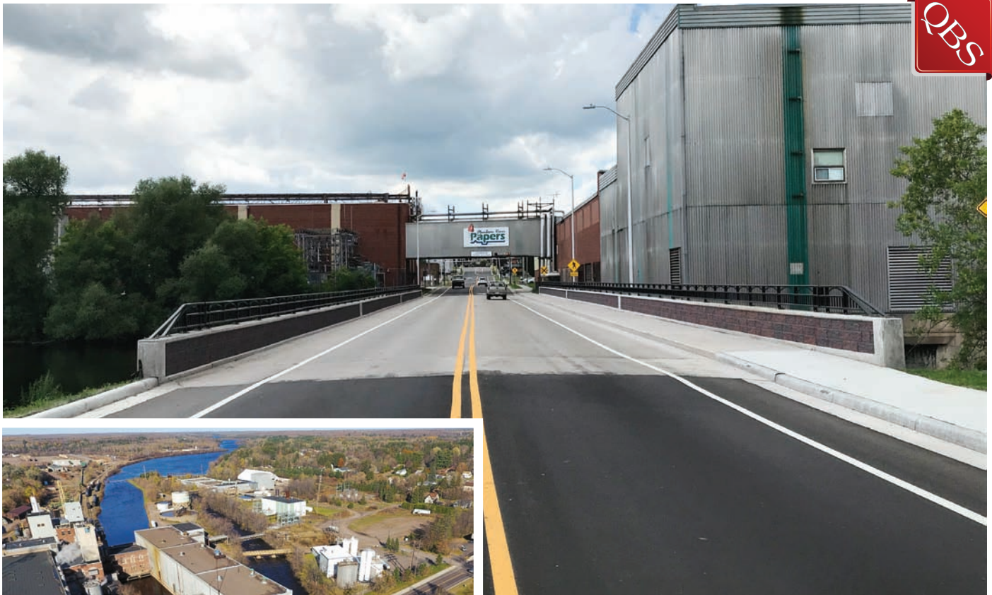
TOP: The new bridge design expands the roadway and provides ample shoulder and sidewalk space. LEFT: The design team navigated close constraints with the paper mill only 10 feet away from the bridge structure and the overhead walkway on one end.
