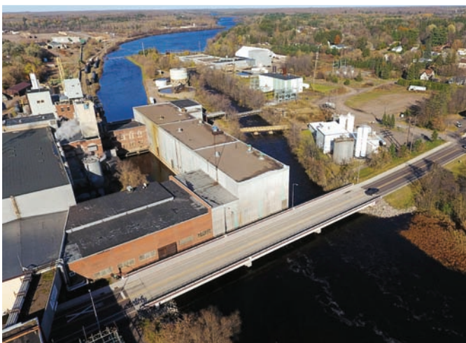
TOP: The new bridge design expands the roadway and provides ample shoulder and sidewalk space. LEFT: The design team navigated close constraints with the paper mill only 10 feet away from the bridge structure and the overhead walkway on one end.
