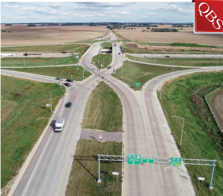
The new interchange uses large curves and relatively straight paths to smooth the transit of OSOW vehicles.
