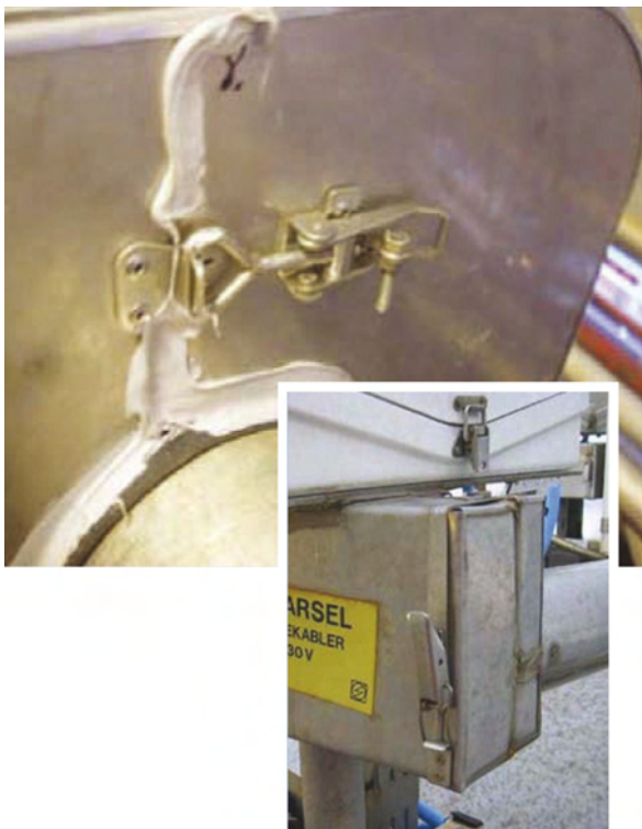
Figure 50: Example locks on insulation cladding
