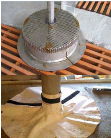
Figure 36: Example of piping and equipment feedthroughs
