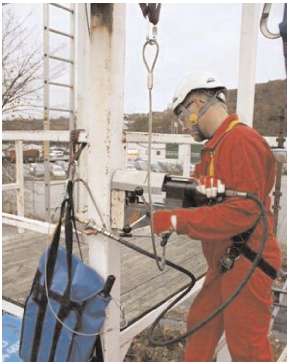
Figure 31: Tools secured against falling
