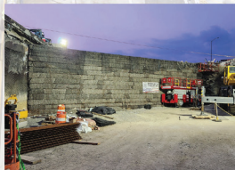
Geogrid retaining wall
