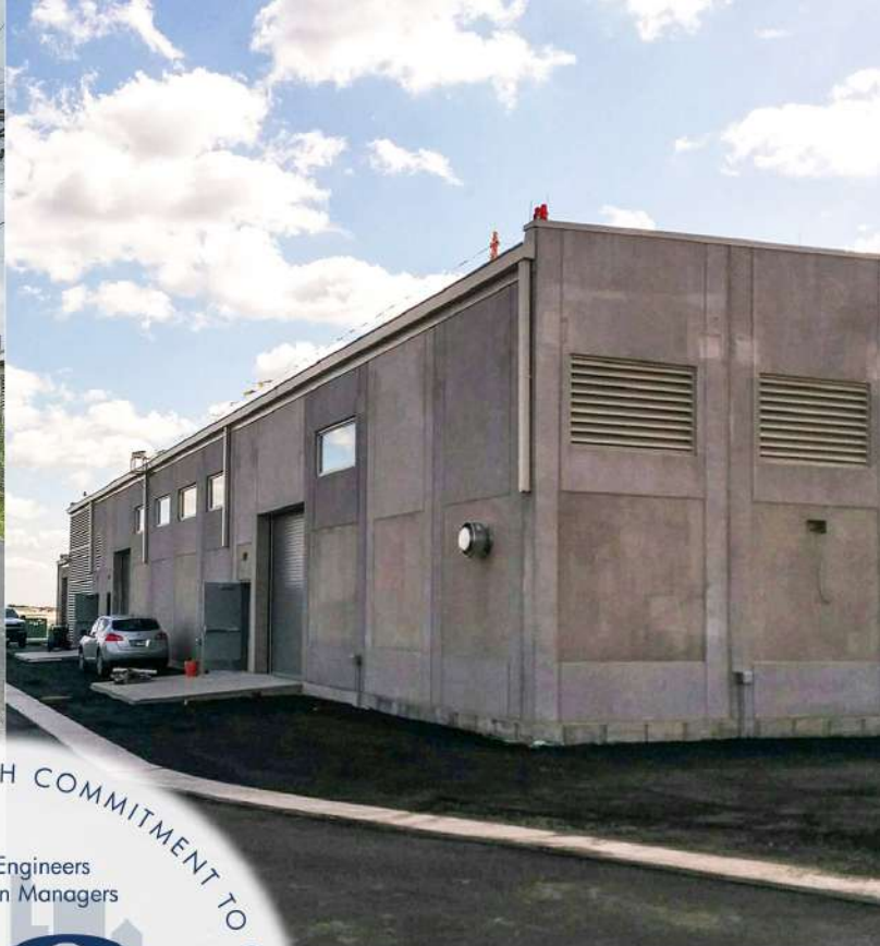
O'Hare International Airport East Airfield Lighting Control Vault 2021 ACEC Special Achievement Award
