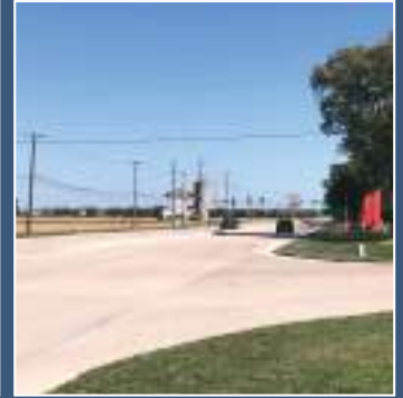
US 34 Widening and Reconstruction
