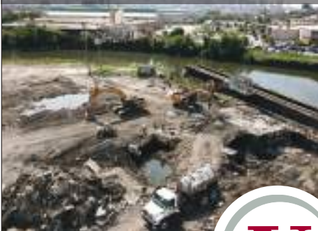
Lincoln Yards North Site Remediation
