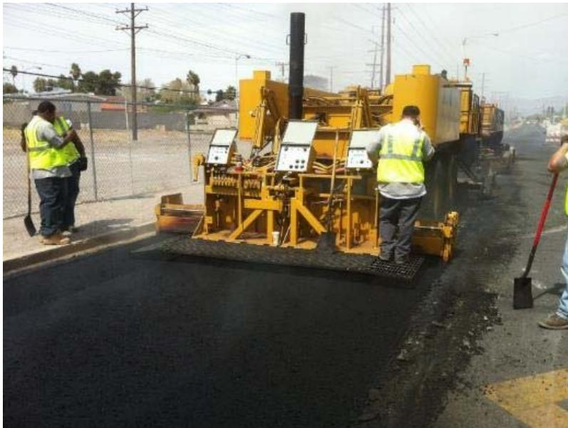
**Figure 15. Laydown Screed (photo courtesy of ARRA)**
