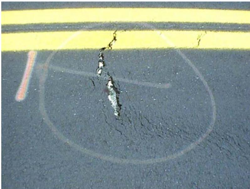
**Figure 19. Cracking and Delamination on CR 315 (Sholar et al., 2002)**
