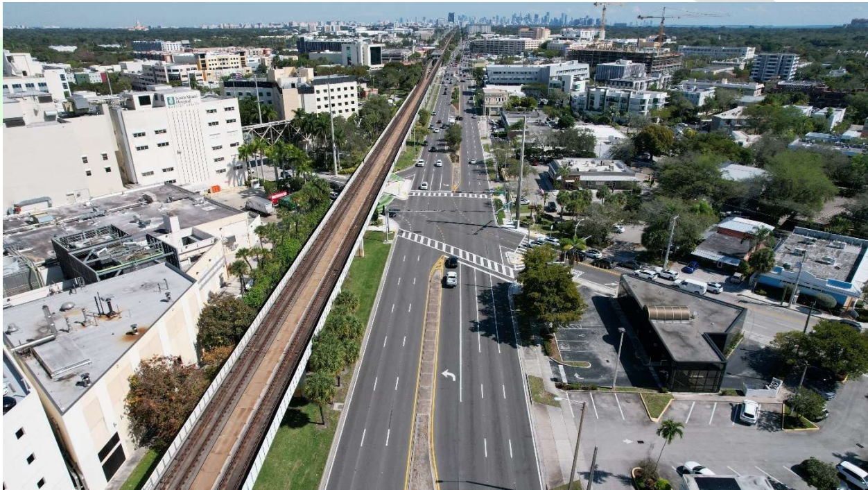
SR 5 (US 1/S Dixie Hwy.) From North of SW 80 St. to South of Riviera Dr.
