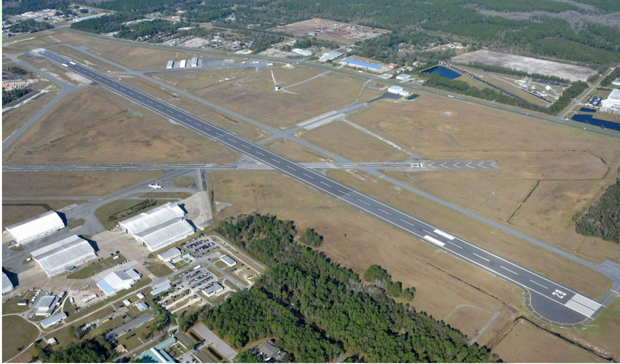
Lake City Airport Runway 10-28
