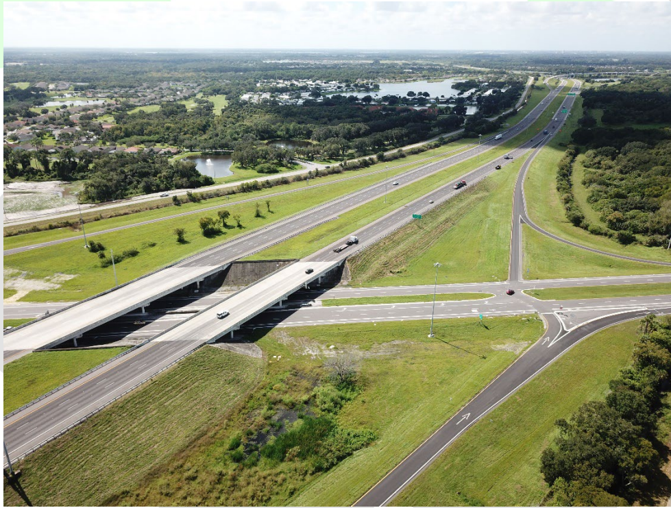
SR 93 (I75) from South of Moccasin Wallow Road to the Hillsborough County Line
