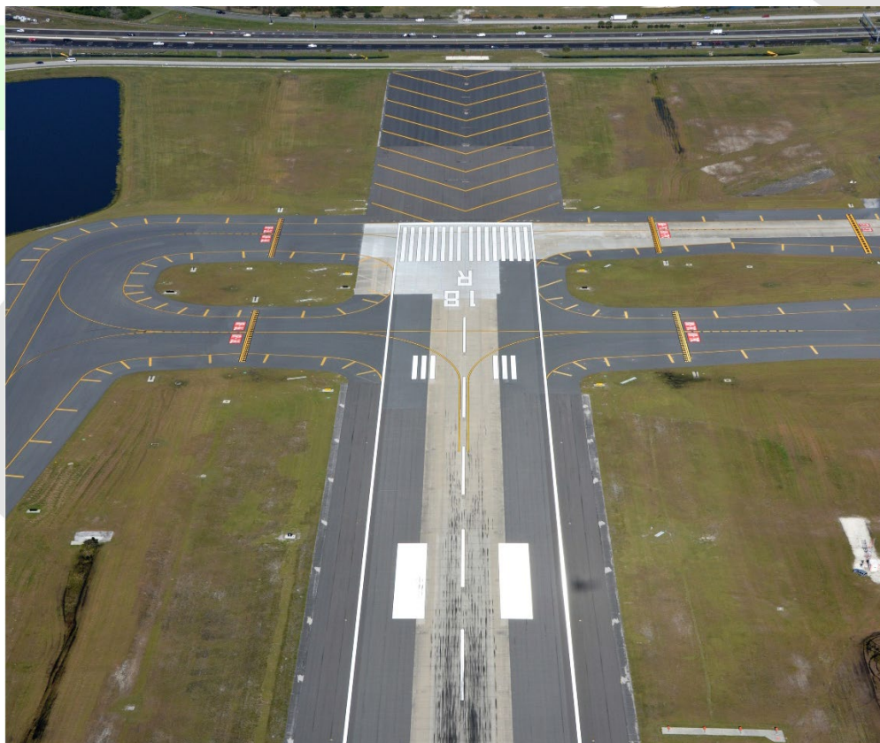
Orlando International Airport Runway 18R-36L
