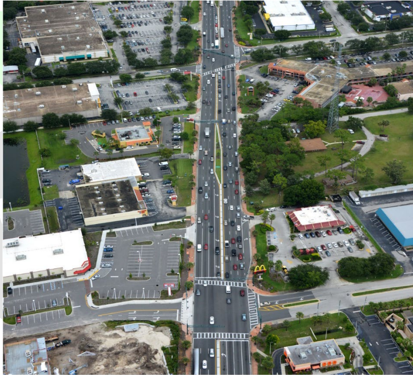
US 441 Orange Blossom Trail (Orlando) from Landstreet Rd. to Oakridge Road
