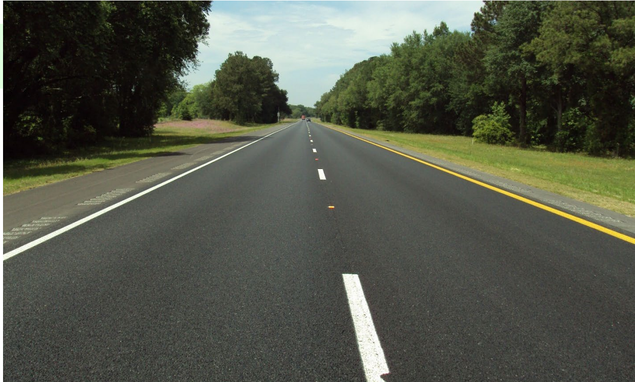
I-10/ SR 8 - From US 90 to US 129, ramps at US 90 And US 129 Interchanges AND US 90 under I-10 overpass
