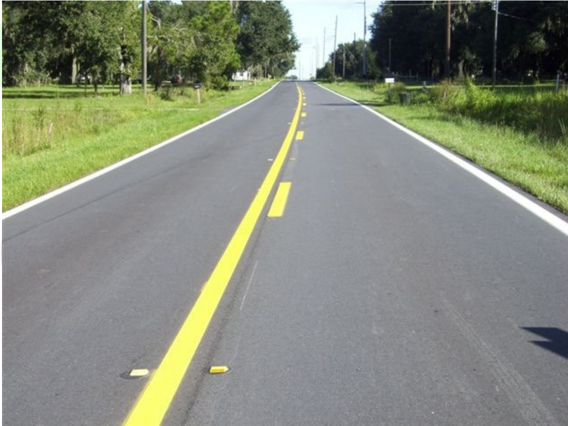
Reconstruction of CR 663 from SR 62, Polk County Line
