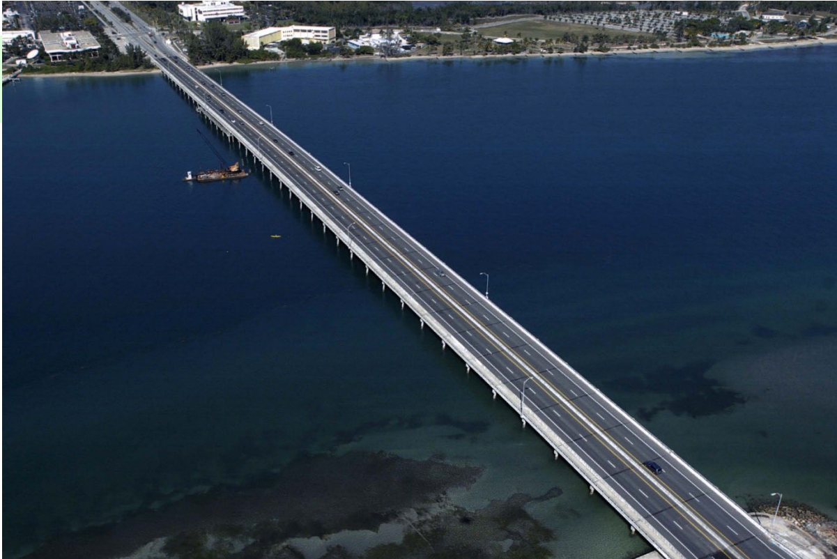
Rickenbacker Causeway on Key Biscayne from the toll entrance to Bear Cut Bridge
