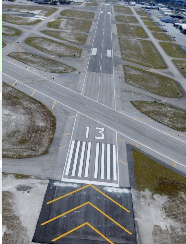
Fort Lauderdale Executive Airport Runway
