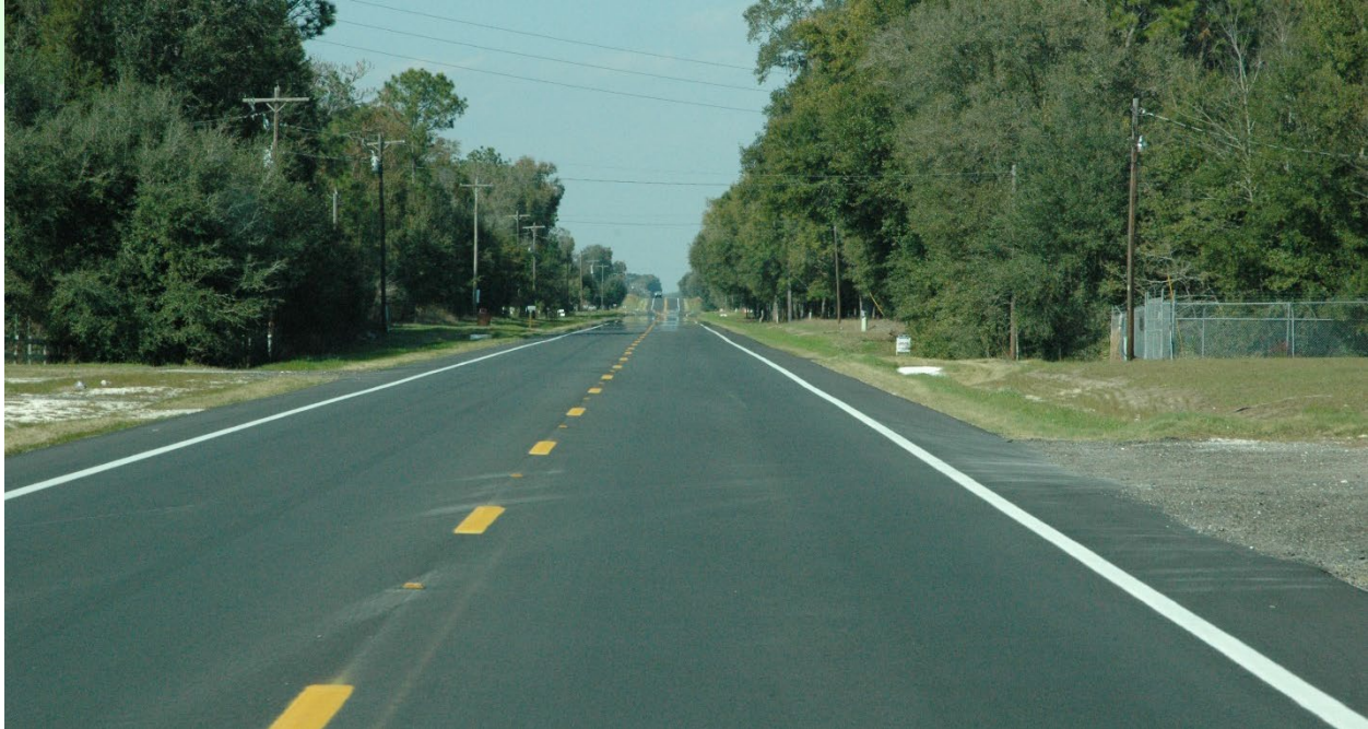
SR 45 (US41) from the Marion/Levy County line to a point north of SW 5th Ave. in Williston, FL
