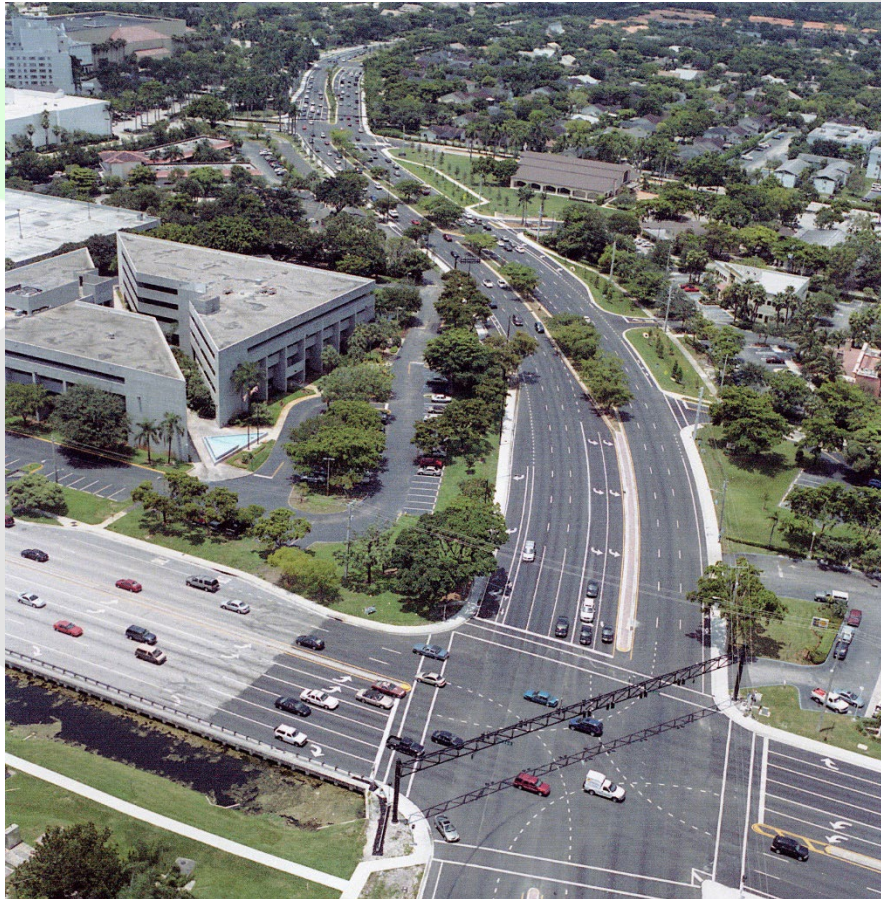
SR 817 (University Drive) from SR 842 (Broward Blvd.) to A Point North of C-13 Canal
