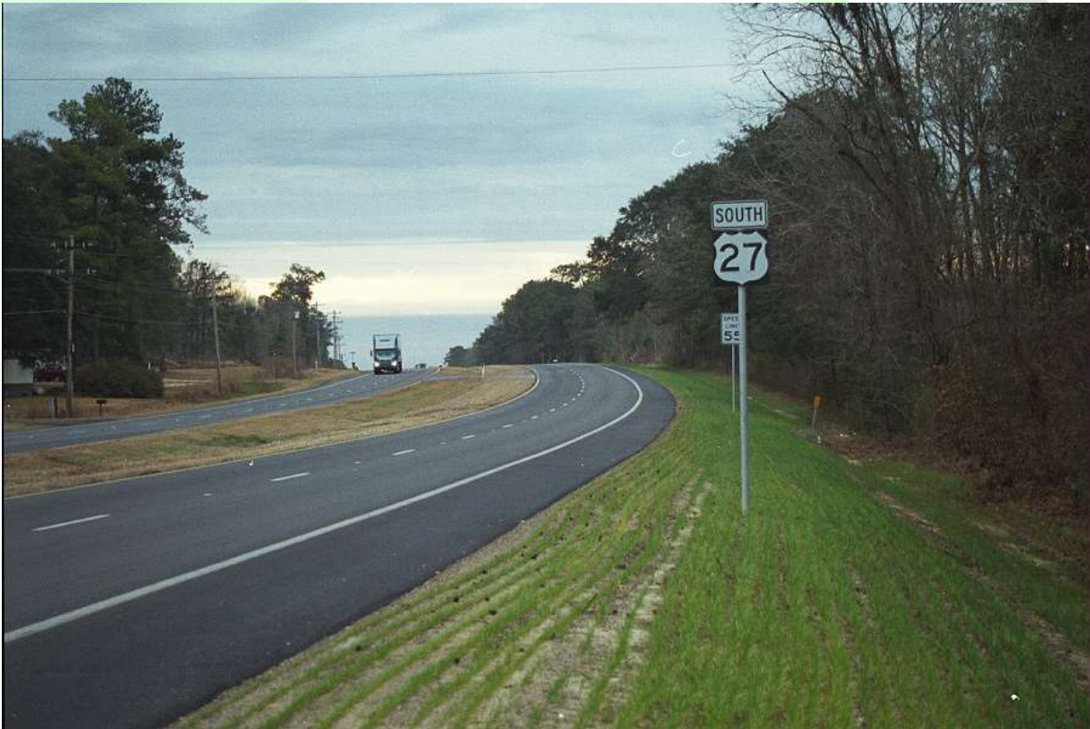
US 27 From Havana City Limits to Ochlockonee River Bridge Gadsden County
