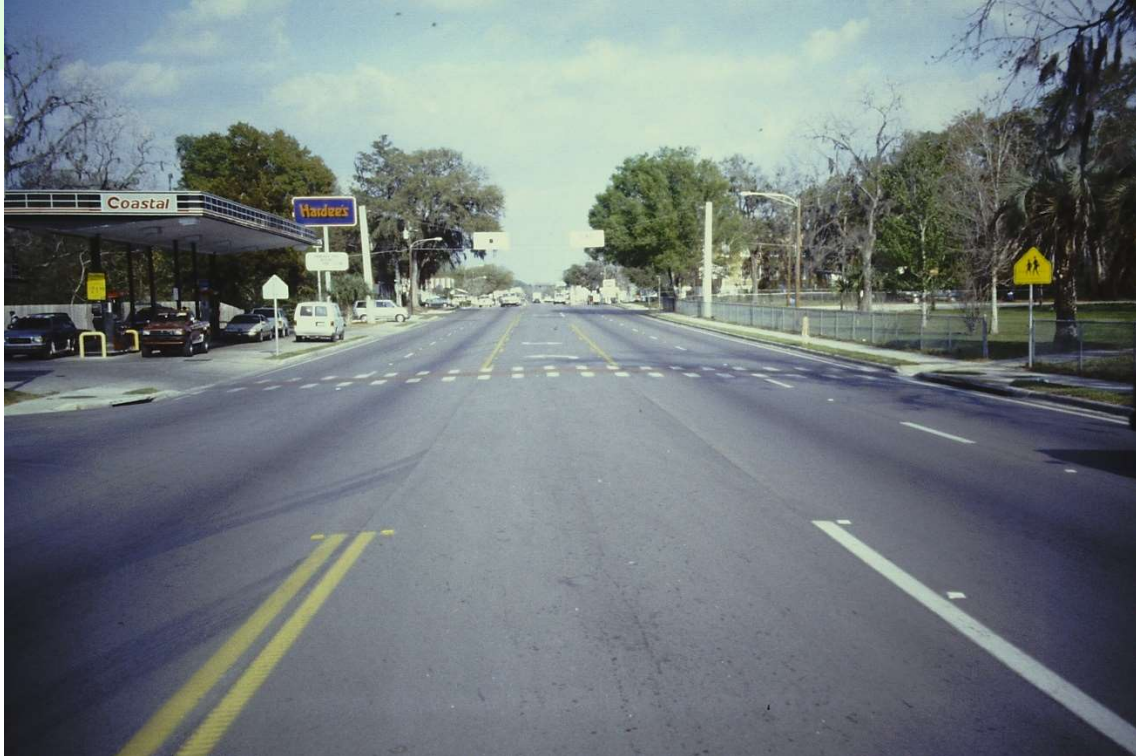
SR 500 (US 27) Noble Ave. in Williston, Florida
