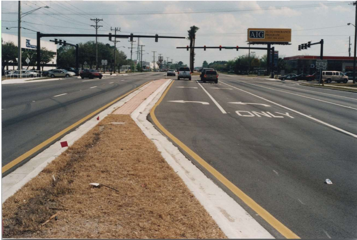
State Road 5 (US 1) From south of the I-95/ US 1 interchange to a point 9.5 miles north Duval County
