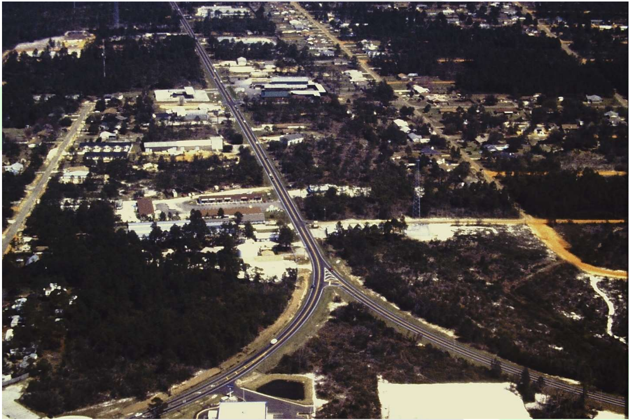
State Road 87 From I-10 to US 98 in Santa Rosa County southeast of Milton
