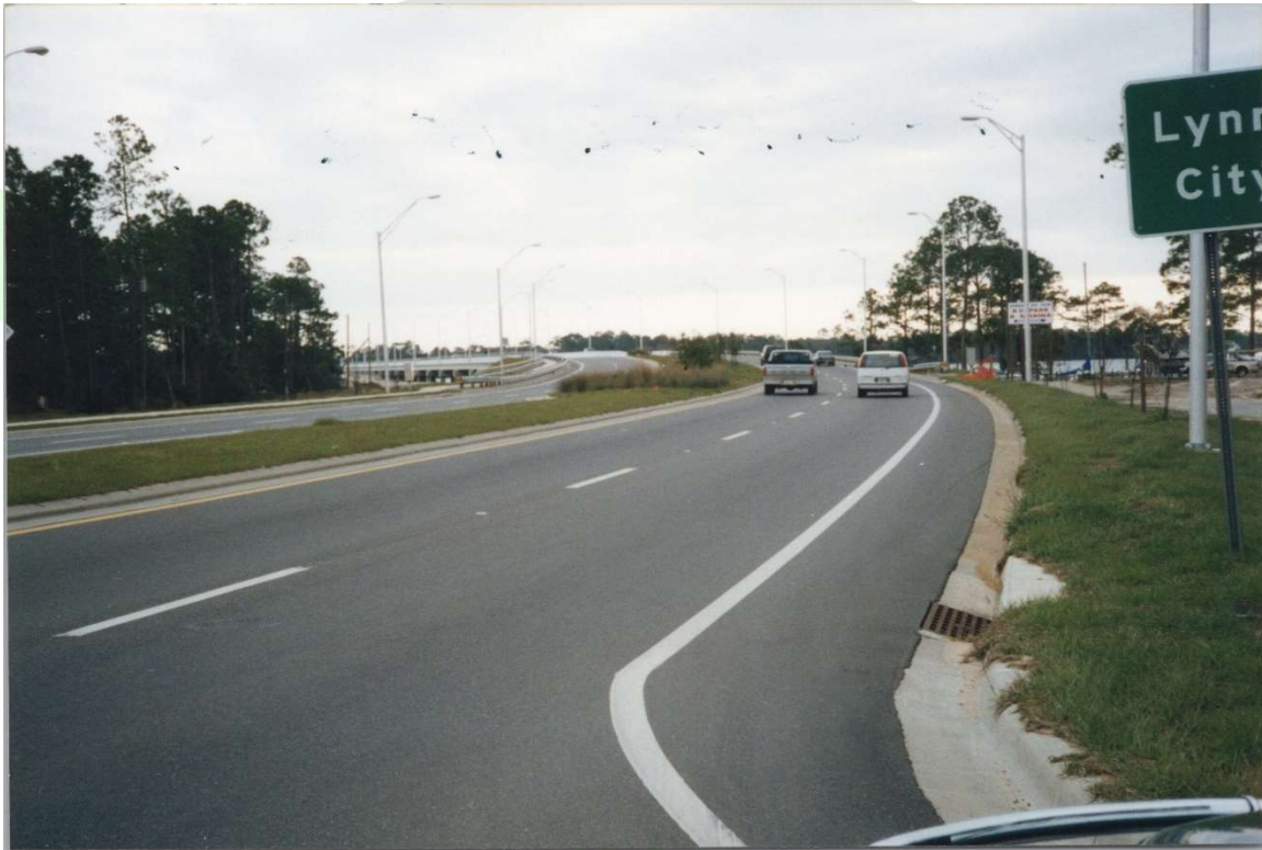
State Road 77, Lynn Haven: Approaches to New Bailey Bridge
