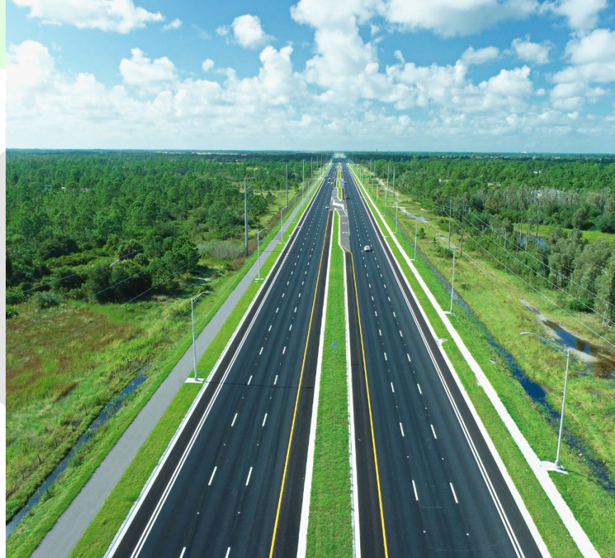
SR 82 from Shawnee Rd. to Alabama Road
