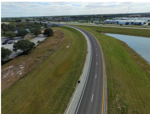
Ranger Construction Industries for their project in Sanford, off ramp from SR 417 North Bound to I-4 East Bound in Seminole County. Tonnage: 383
