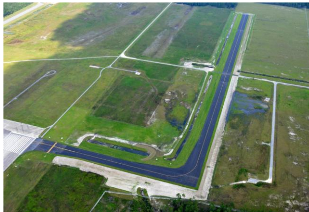
Duval Asphalt Products for their project on the Cecil Airport East Development, Taxiway E in Duval County Tonnage: 10,440
