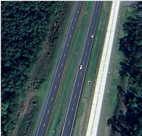
Field Trials (e.g. Test Road on US 301)
