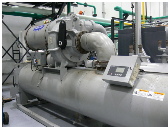
Figure 17. Low-Pressure Chiller.
