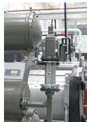
Figure 18. Rupture Disc.
