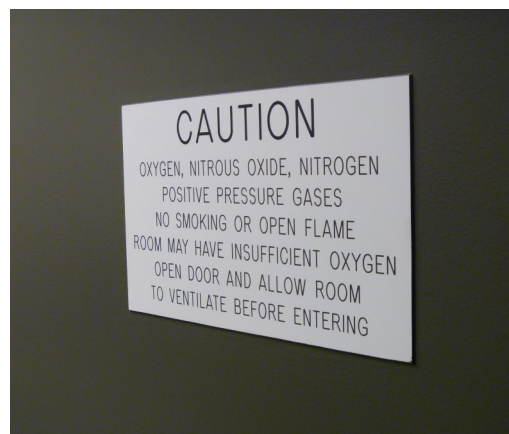
Figure 19. Equipment Room Wall Plate.
